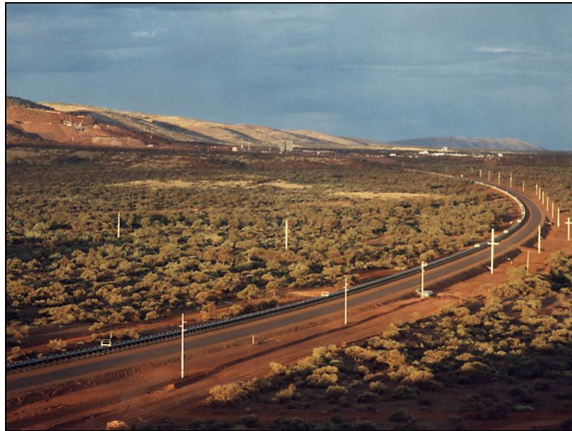
Figure 23 – Channar Overland Conveyor System
