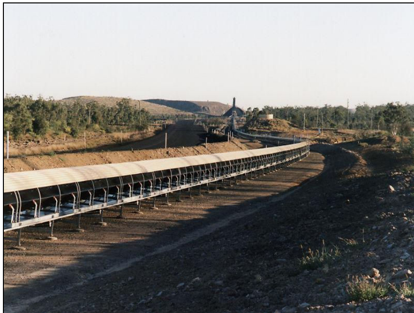
Figure 24 – German Creek Overland Conveyor
