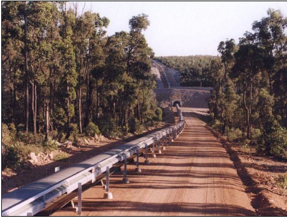
Figure 31 – Muja Overland Conveyor System
