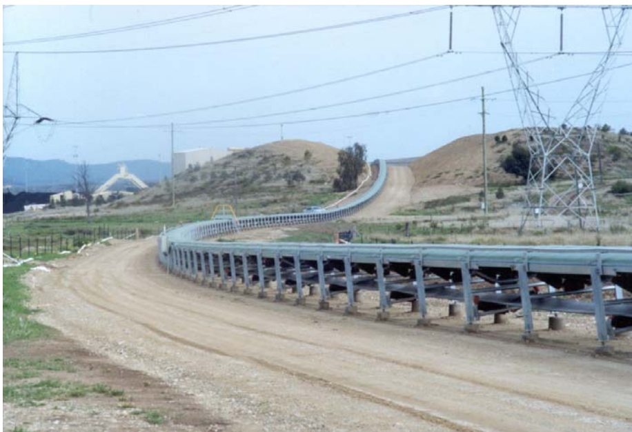
Fig. 1 Warkworth overland negotiating obstacles using a low profile hood cover - Australia
