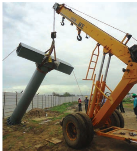
Erecting the First Bent.
