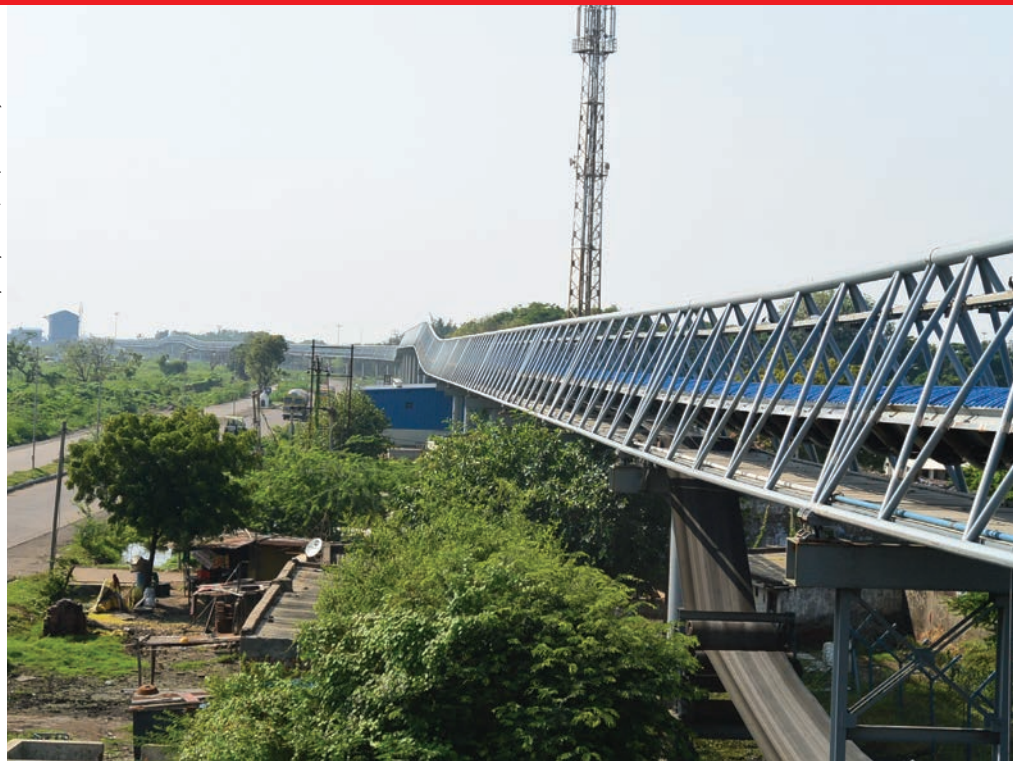
Maintenance trolley that allows maintenance personal access to the conveyor.
