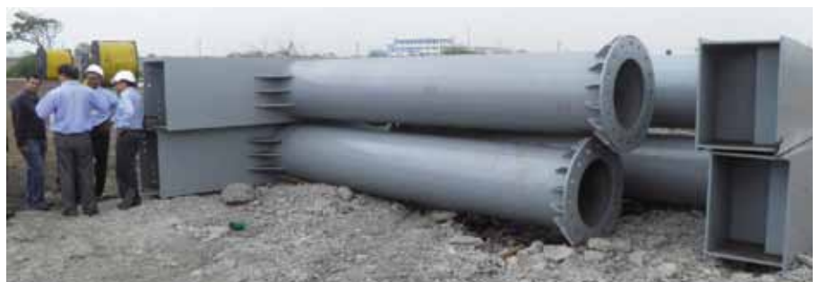
Fig. 10: Bent laydown yard.
