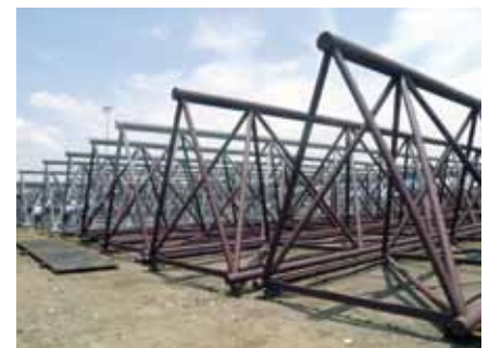
Fig. 4: Laydown yard of the tubular triangular conveyor galleries.
