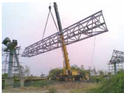
Fig. 12: Installing a gallery.
