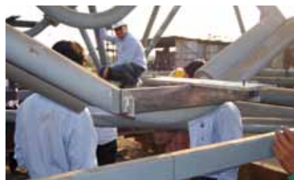
Fig. 5: Custom idler jig for positioning the idlers in horizontal curves.
