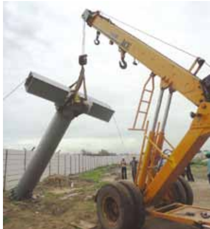
Fig. 11: Erecting the first bent.
