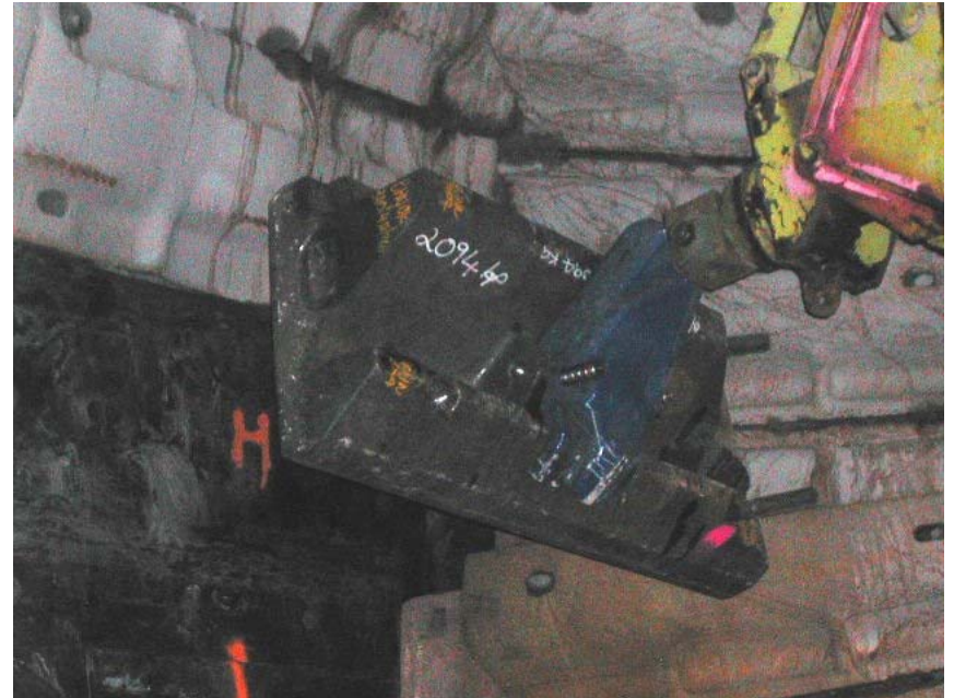
Figure 7: Trial castings installed in the 40 foot Diameter SAG Mill
