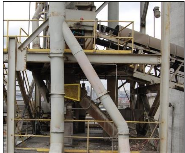
Figure 9. Ash Grove Cement Company, Seattle Plant, Original Design at TT6
