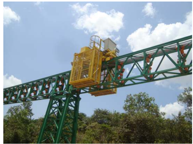
Figure 4. Brazil Itaqui Pipe Conveyor: Box Truss with Trolley
