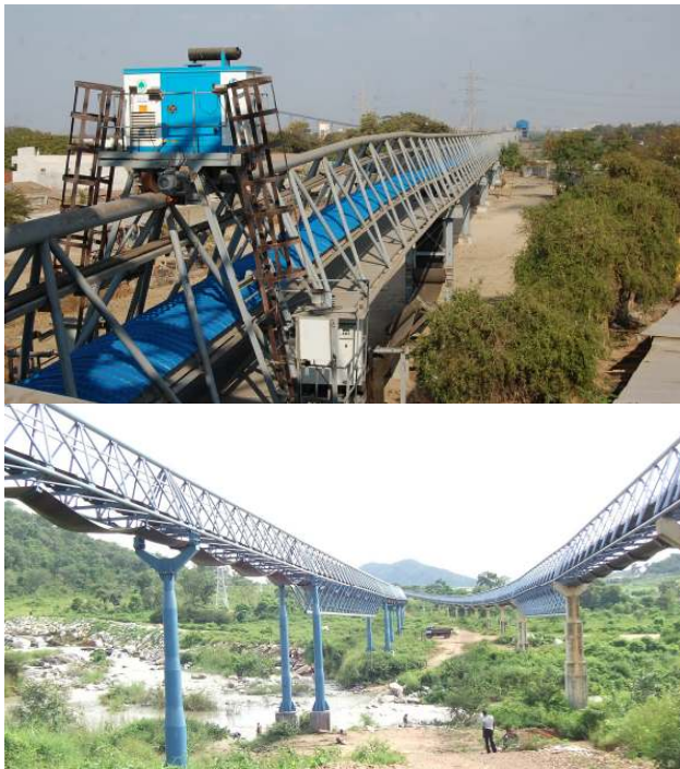
Figure 3. Triangular Truss with Trolley. Top: India Dahej 6000 T/H coal conveyor; Bottom: Nigeria Dangote 2400 T/H (right) and 3500 T/H (left) limestone conveyor
